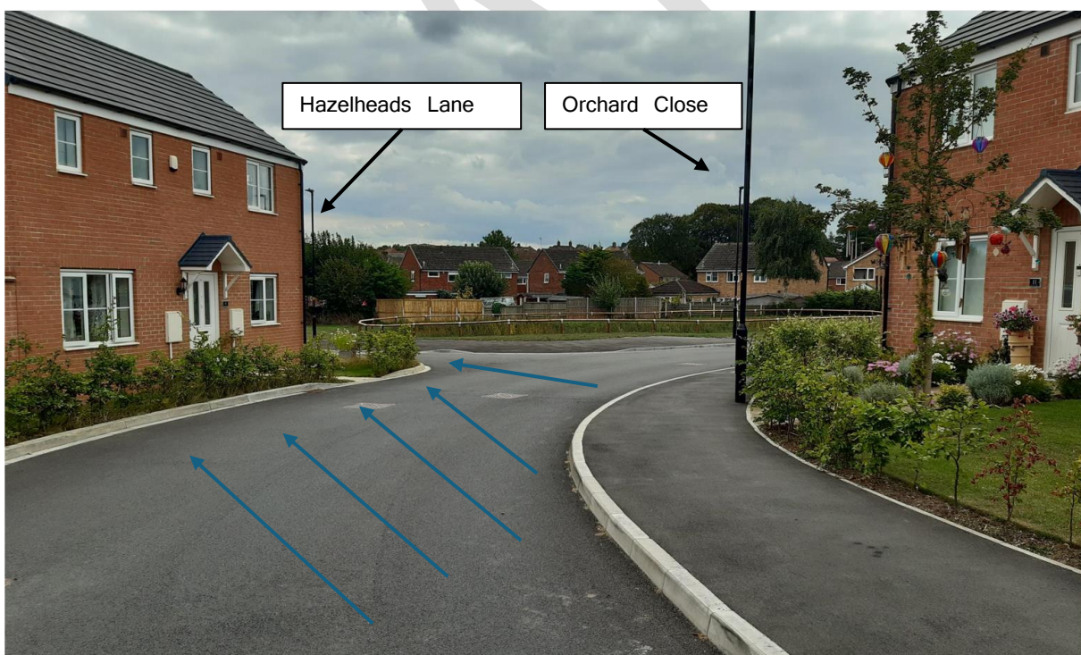
Figure 11: Carriageway Crossfall Bramley Way
